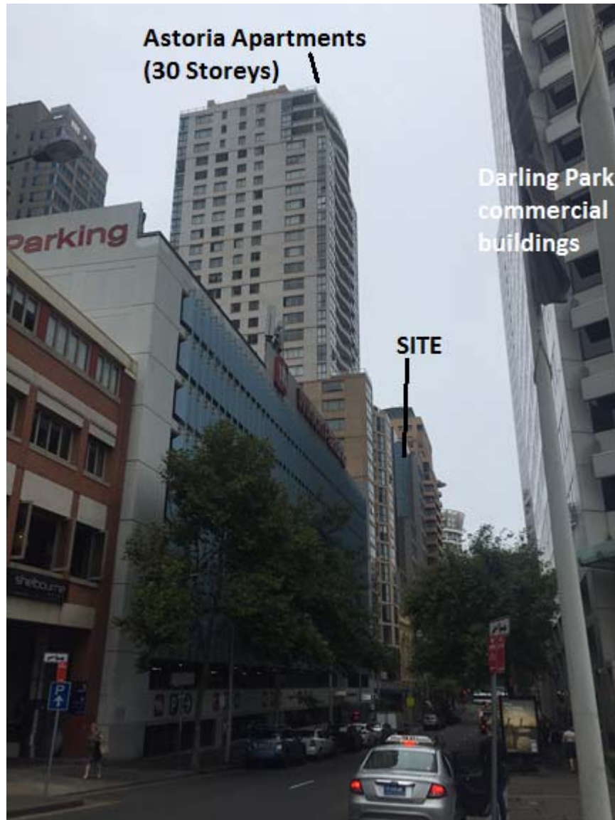
Figure 8: Context view – View looking south down Sussex Street
